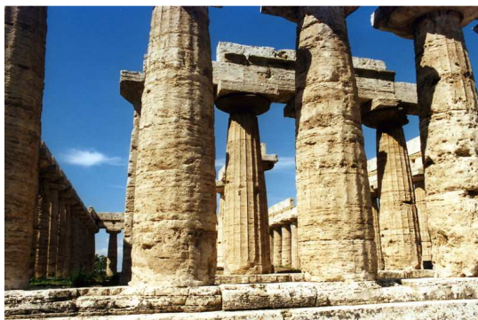
Fig. 1 Entasis- characteristic curvature of Doric columns
